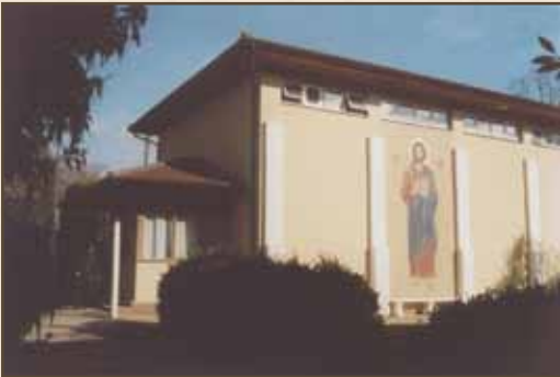
St Silouan's Church.
