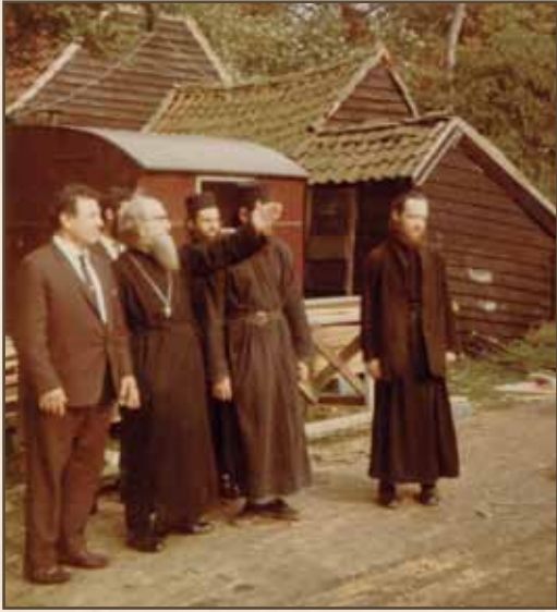
Studying the site for future buildings.
